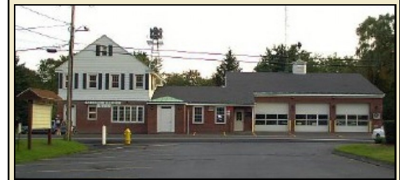
Station #1 126 Maple Ave. Selkirk
